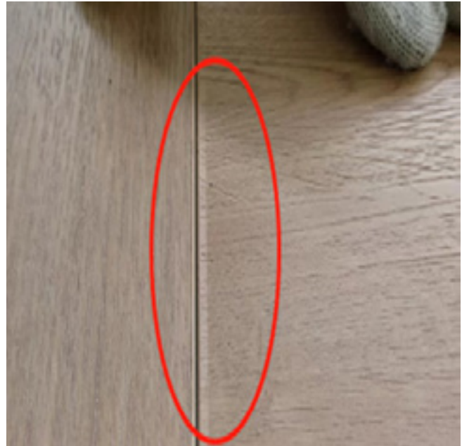
Here, the board has been broken as the mallet was used when the board was still lifting
