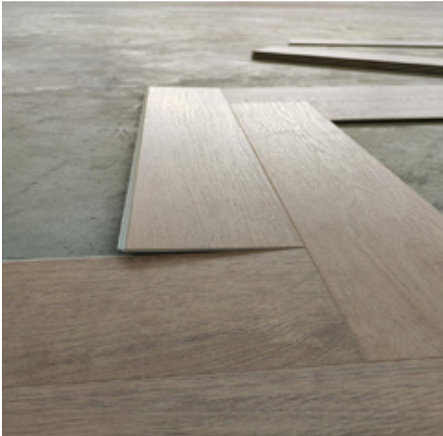
Here, the board is still lifting
