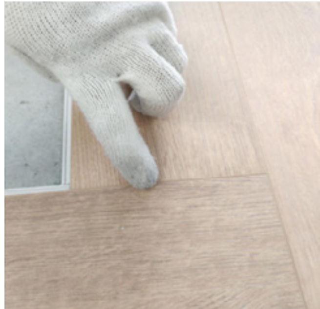
Checking the tongue touches the groove
